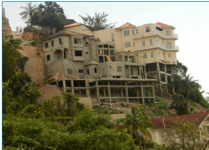
Plate 3.1: Example of poor hillside construction practice
