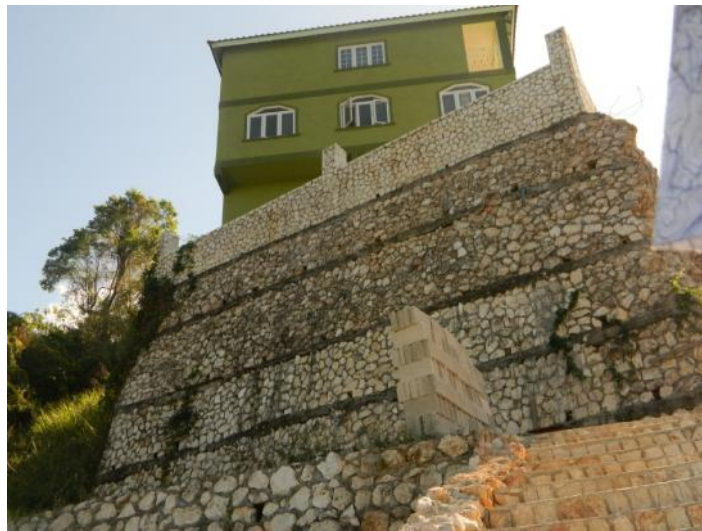
Plate 4.2: Height of this retaining wall is approximately 12m (39.4ft) and is used to support deep fill. This is not recommended. Stepped retaining wall is normally the preferred option.
