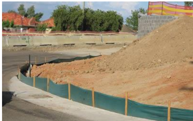
Plate 6.4: Example of silt fence to prevent sediments from leaving the site
