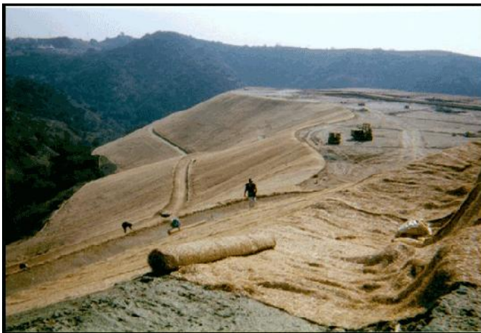
Plate 6.2: Example of erosion control mats to protect hillsides from erosion
