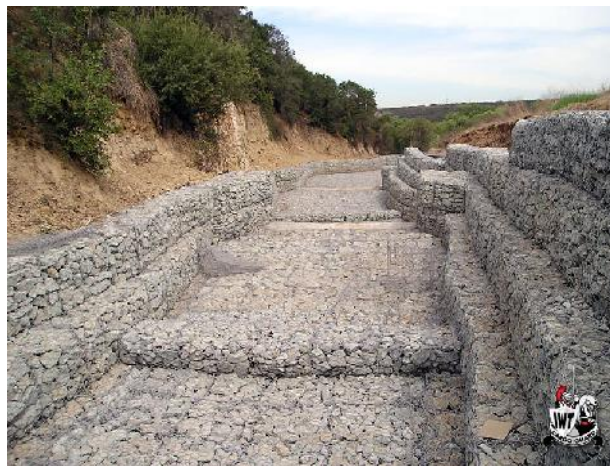
Plate 6.5: Reno Mattresses and Gabions used for erosion and sediment control.
