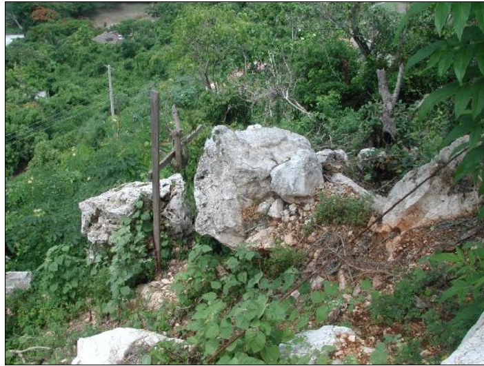
Plate 4.1: Loose boulders located on slopes are susceptible to rock falls from severe rainfall or earthquake events. These must be removed during site preparation.
