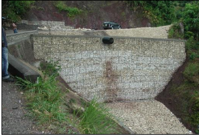
Plate 6.1: Gabion baskets as a method for slope and erosion protection for roadway in Buff Bay Valley, Portland
