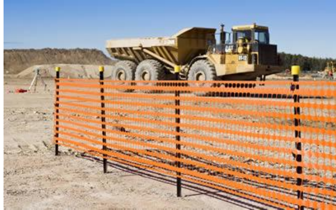
Plate 6.3: Silt Fence for sediment control
